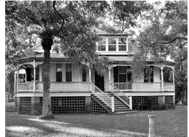
Structural supports take into account the location of prominent features and repeat vertical elements. Shown here is 116 Ballentine Street (demolished), circa 1880, Bay St Louis.
