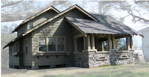
Significant façade components such as major masonry features require special consideration.
